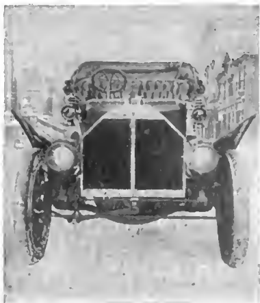
FRONT VIEW OF DUPLEX RADIATOR.
